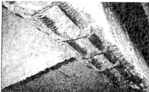
Fig 5. Debonding and corrosion of longitudinal bars and stirrups of reinforced concrete bridge beam
