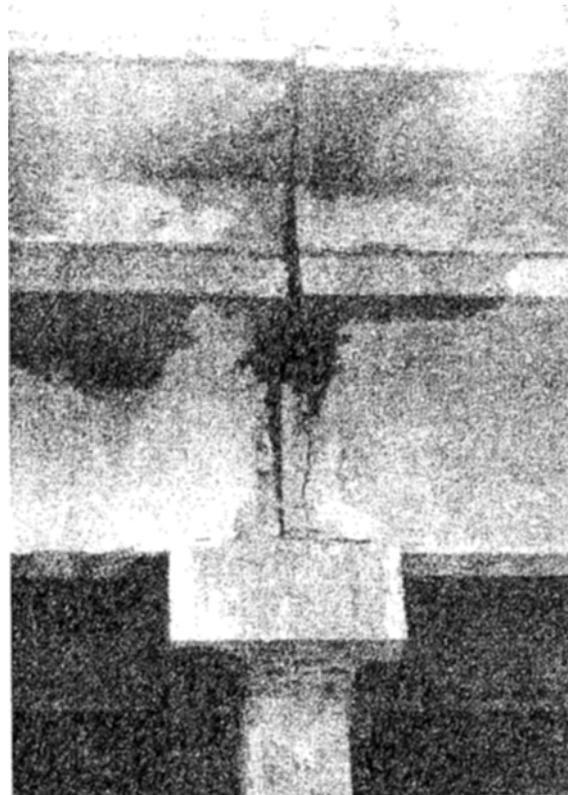
Fig 9. Deterioration of edges of beams and cap of pier due to leakage of expansion joint
