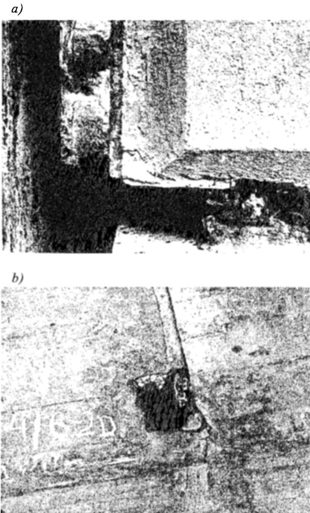
Fig 13. Corrosion of exterior anchors of tendons: a) – at the edge of simple beam; b) – at the joint of segmental post-tensioned bridge beam
