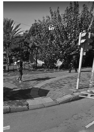
Figure 12. Tactile paving and sidewalk ramp in Antalya ( https://www.google.com/maps/@36.8588256,30.7922636,3a,75y,301.24h,74.45t/data=!3m6!1e1!3m4!1shYcV6ERkDBxi2UHlojzoYw!2e0!7i13312!8i6656 )
