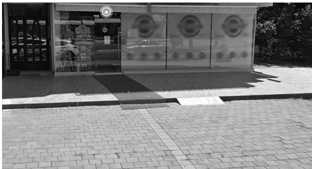
Figure 10. Entrance ramp for a pharmacy in Antalya ( https://www.google.com/maps/@36.8742525,30.6264924,3a,75y,97.87h,86.42t/data=!3m6!1e1!3m4!1sSJldvuOML2tYe7UIFkqKqA!2e0!7i16384!8i8192 )
