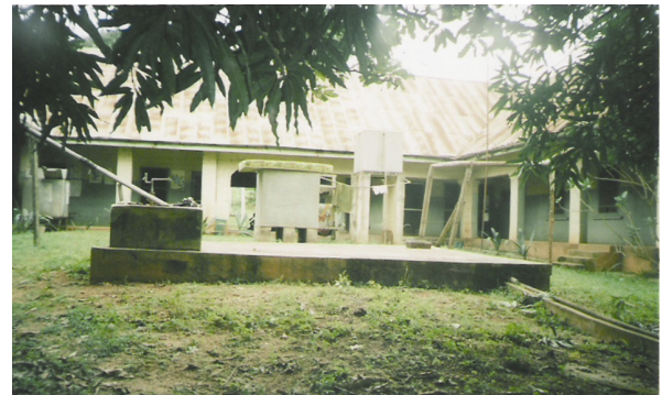
Fig. 2. The leprosarium with centralized concrete rain-water harvesting tank and 3 galvanized iron tanks for water storage
