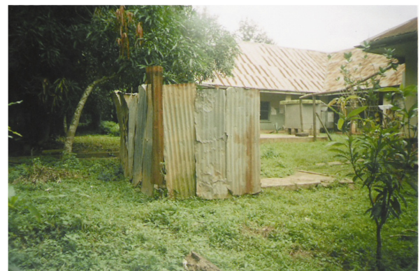
Fig. 4. Back view of an improvised bathroom for the leprosarium. Wastewater percolates into the soil
