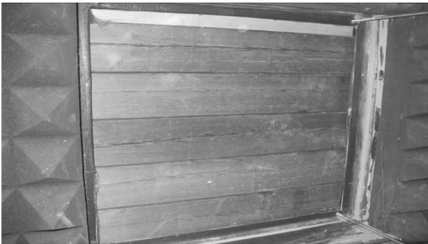
Fig. 4. View of an element of the log wall, 15 cm wide, assembled in the noise suppression chamber
