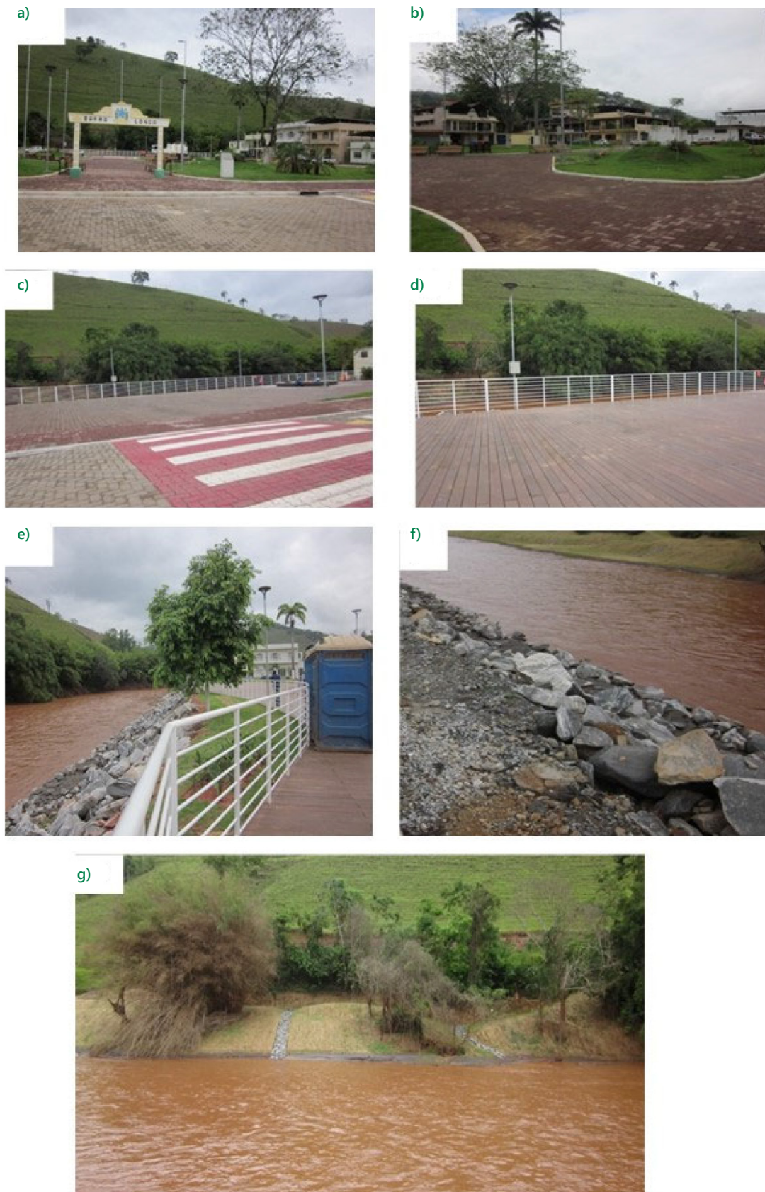
Figure 6. Rehabilitation of the Lino Mol Square (a and b); coverage of the riparian area with a wood deck (c, d and e), stones (e and f) and plant-derived fibre mats (g)
