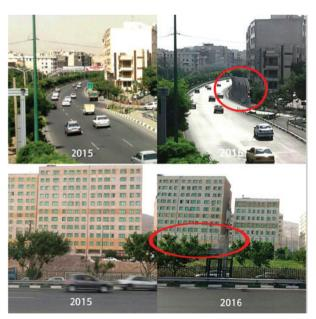
Figure 10. Before & after installation of noise barriers in some measurement points
