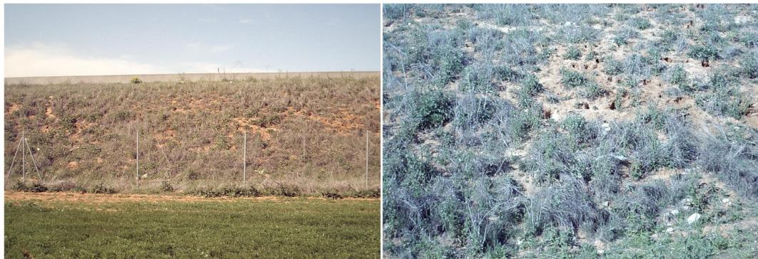
Figure S9. A3 motorway. Rabbit warrens in embankments (2002) may produce a significant loss of herbaceous cover
