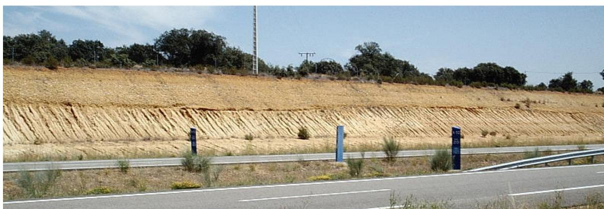
Figure S15. A52 motorway (Zamora, NW Spain, 2002). Differential erosion on a roadcut; the lower part is more eroded
