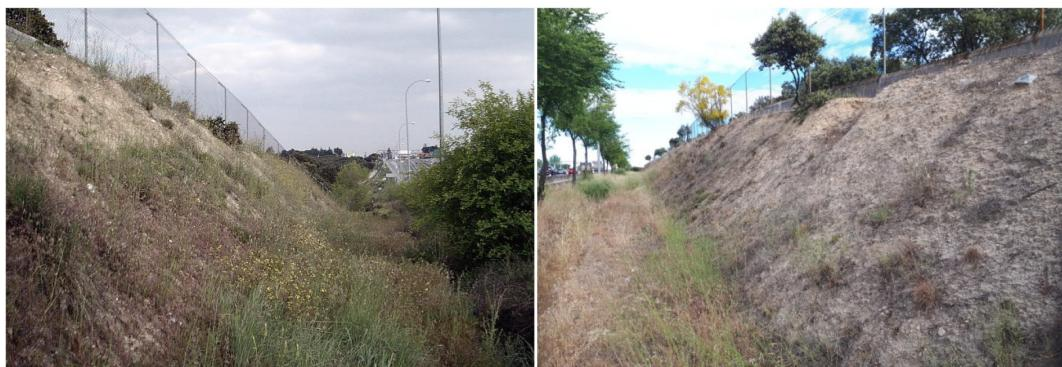
Figure S10. A6 motorway. Cutting in arcoses. Left: 2002. Right: 2019. The evolution has been regressive
