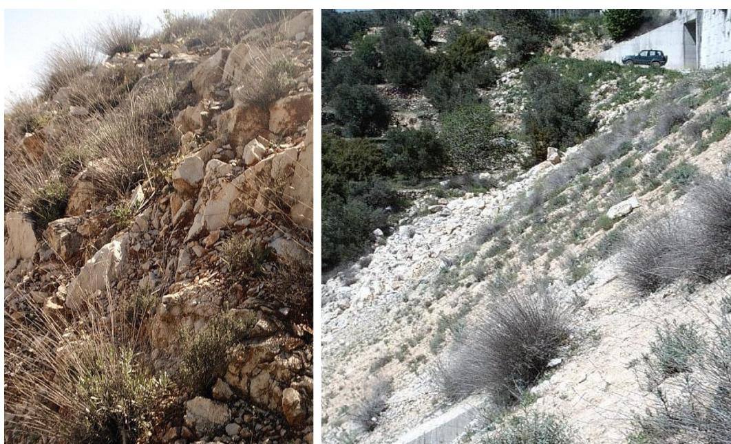
Figure S8. A3 motorway. Left: Rock cutting (2002); the plants observed are *Lavandula latifolia*; seed of this species was included in the hydroseeding, which has allowed the colonization of the slope.
