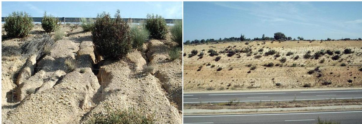
Figure S13. A52 motorway (Zamora, NW Spain, 2002). The slopes have been planted, but not hydroseeded. As a result, erosion problems are intense. Left: Embankment. Right: Cutting
