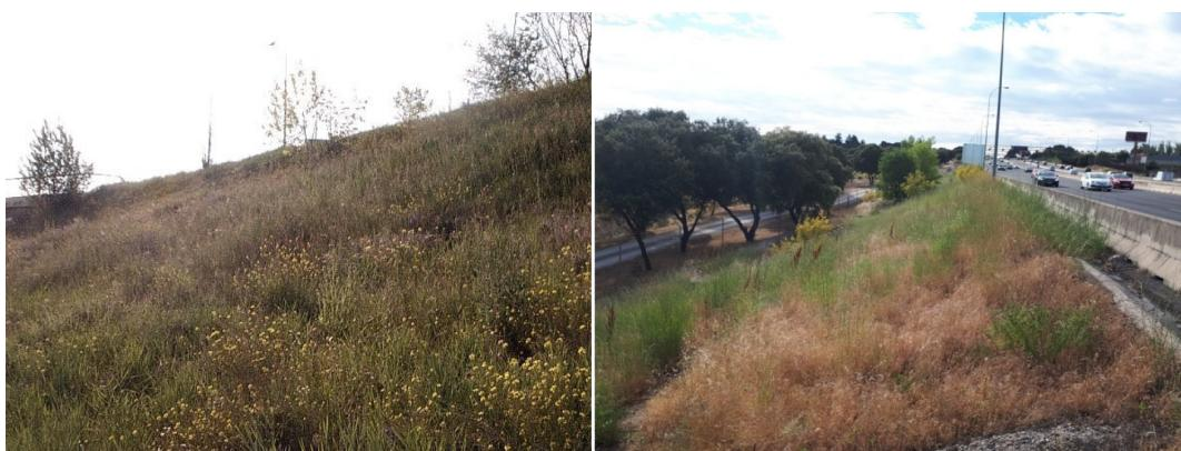
Figure S11. A6 motorway. Cutting in arcoses. Left: 2002. Right: 2019. The evolution has been regressive
