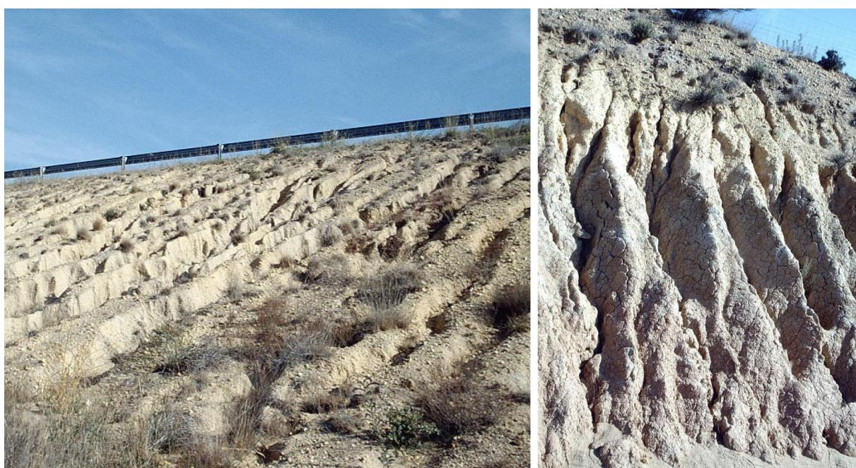
Figure S14. A52 motorway (Zamora, NW Spain, 2002). Erosion in slopes not revegetated. Left: Embankment. Right: Cutting
