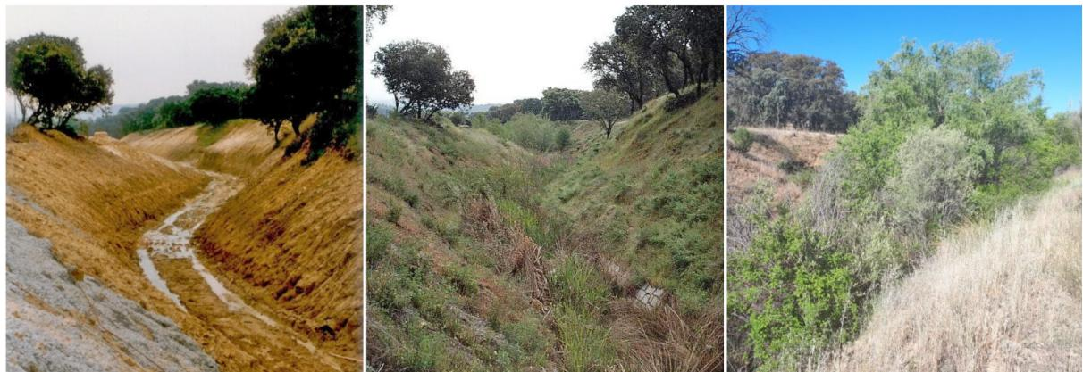
Figure S3. M40 motorway. Creek channelled during road construction. It was revegetated like the roadslopes, with topsoil, hydroseeding and plantations. Left: 1994. Centre: 2002. Right: 2019
