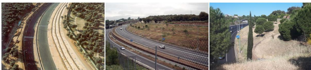
Figure S2. M40 motorway. Cutting. Left: 1994. Centre: 2002. Right: 2019. The slope is frequently mown, making impossible the development of shrubs, and limiting the natural evolution of the slope
