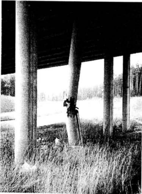
Fig 2. Collision damage of reinforced concrete edge beam (a) and pier column (b) of highway viaduct, and of main beam of the suspension steel footbridge (c)
