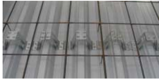
Fig 10. Shear connectors Hilti Stripcon fastened to the steel beam before concreting
