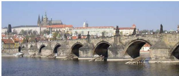
**Fig 1.** Charles Bridge with 16 arches and a clear span of 16,62 m to 23,38. The overall bridge length is 515,76 m and it is 9,4 m wide. The dimensions of massive stone piers at the arch footing range between 8,5 m and 10,84 m by 24,0 m to 25,0 m. Pier heads have been “sharpened“ against the water stream at an angle of 65°. The bridge construction started in 1357 and was completed in 1406
