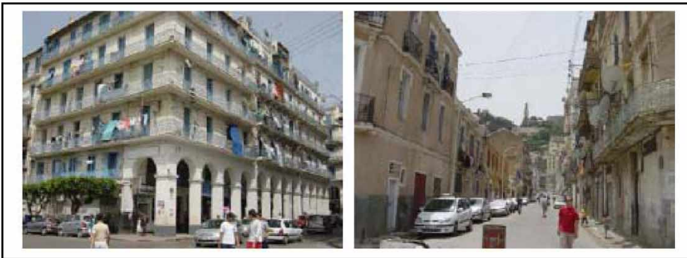
(1) Houses and shops Masonry buildings
