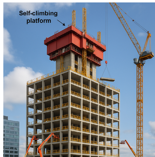
Figure 15. Schematic of self-climbing platform operation in high-rise construction
