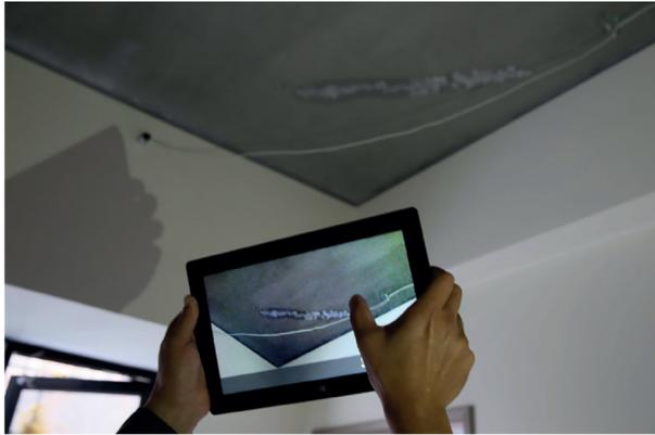
(b) On-site quality engineer marked the defect in the photo and BIM models and entered the defect records in the tablet
