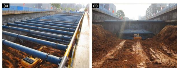
Fig. 5. Working site of the excavation of the Mingdu Station: (a) steel support; and (b) foundation pit
