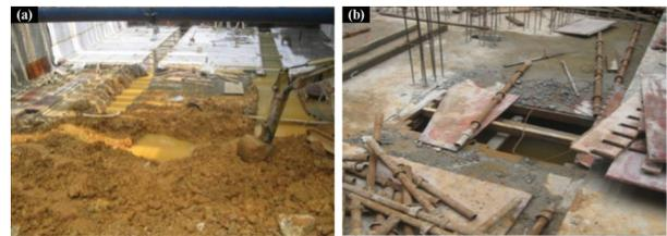
Fig. 8. Risk event of water gushing at the Mingdu Station: (a) location of water gushing; and (b) a precipitation well
