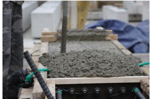
Fig. 8(b). Concrete cast
