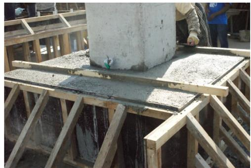
Fig. 8(c). Fabrication of foundation
