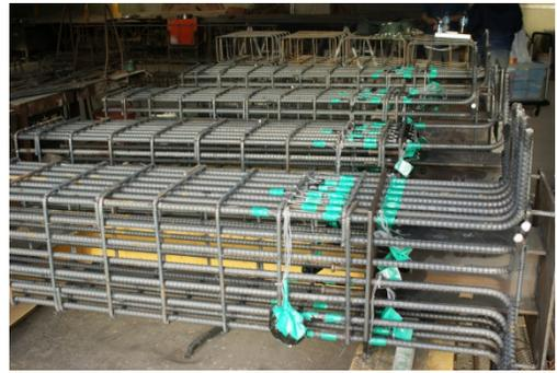
Fig. 8(a). Assembly for re-bars and steel sections
