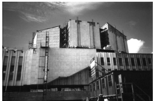
Fig 10. Alvar Aalto, Finlandia talo (Finlandia Congress and Concert Hall in Helsinki, 1969–1975 during changing of marble plates, 1998
