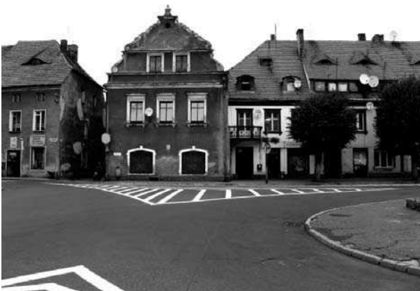
Fig. 4. Frontage of market square in Prochowice, to the left from a house of 1588
