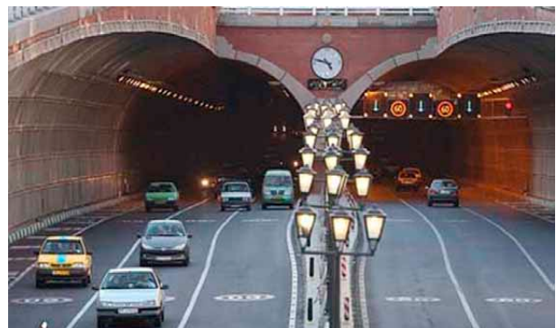
Fig. 3. Tohid tunnel (Fars News Agency 2015)
