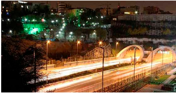
Fig. 1. Resalat tunnel (Hamshahrionline 2015)
