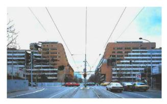
Fig. 4. The Army Headquarters after the 1999 bombardments and redefined recognisability. The Building A with significant damage and the Building B with slight damage and demolished entrance pavilion (on the far right). *Source*: Kovačević (2001).
