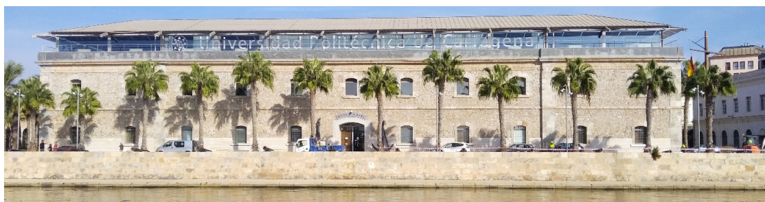
Figure 7. The CIM building, hosting the UPCT Department of Architecture (ETSAE) and the Naval Museum (source: author's personal archive)
