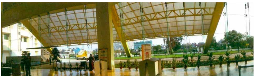
Inviting entry lobby and porch to hospital
