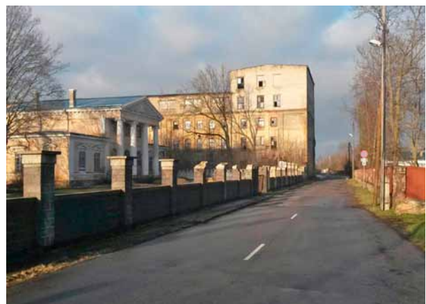
Fig. 10. The former flax spinning mill and Villa Medem Source: author's photo, 2015
