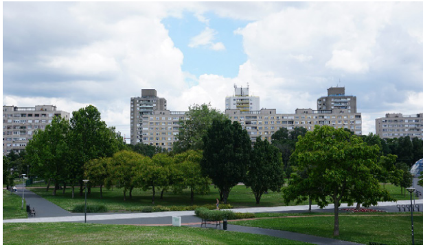
Figure 12. Kelenföld' central green park, the Bikás, 2018 (source: author)
