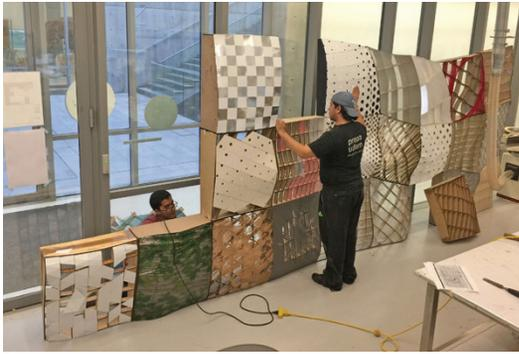
Figure 5. Mounting the cells into the whole installation assembly of the parametric wall
