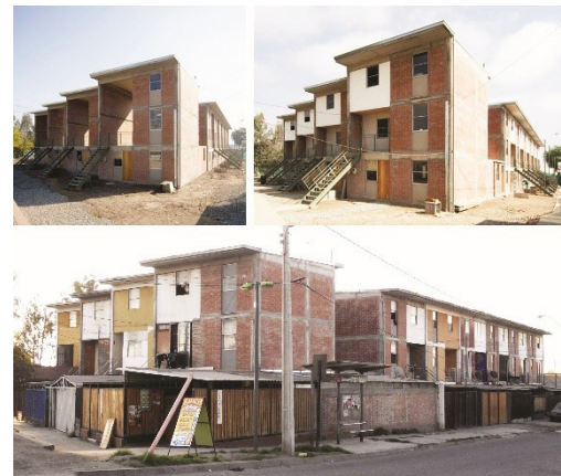
Figure 2. (above) Base house of Lo Espejo, Elemental Architectural Office, 2006 (source: http://divisare.com/projects/280780-ELEMENTAL-Alejandro-Aravena-Lo-Espejo ); (below) customised houses of Lo Espejo, 2015 (source: the author)
