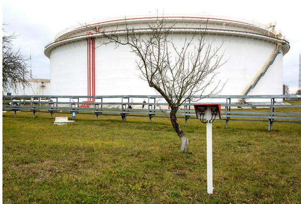
Figure 2. Ground vertical cylindrical steel welded tank with a nominal capacity of 75.000 m<sup>3</sup> with a floating roof and a double wall of the LODS “Brody” company
