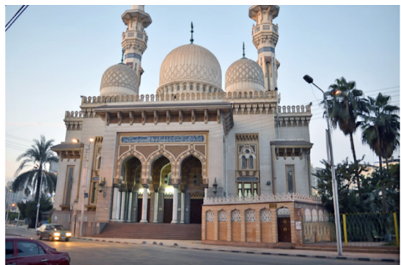
Figure 1. El-Nasr Mosque façade, Mansoura city, Egypt (the studied historical building)
