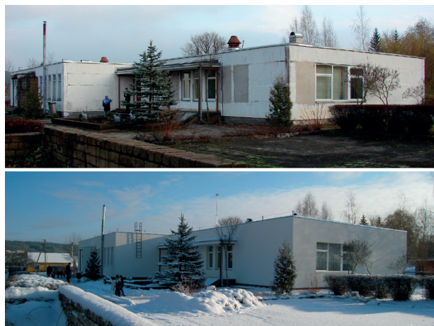
Fig. 2. Nursery school in Semeliškės before and after renovation
