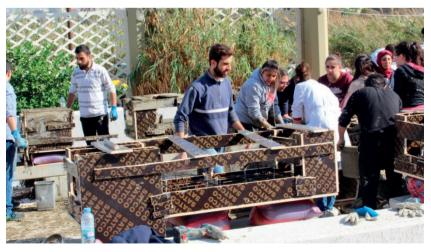
Figure 9. The construction phase of the street furniture: seating benches and flower boxes. It was constructed in-house on Beirut Arab University Tripoli campus with the help of Beirut Arab University level three architecture students (source: created by authors)
