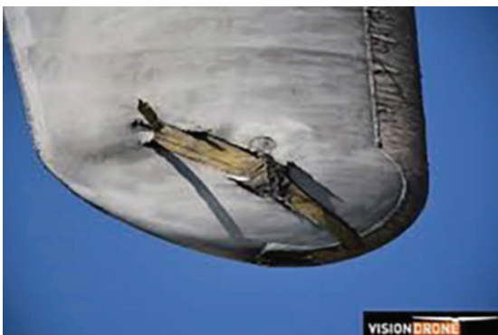
Figure 2. Damaged leading edge of a wind turbine blade (Motion, 2017)
