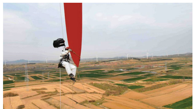
Figure 1. Inspection of a wind turbine conducted using the rope descendent technique (Nurm, 2017)
